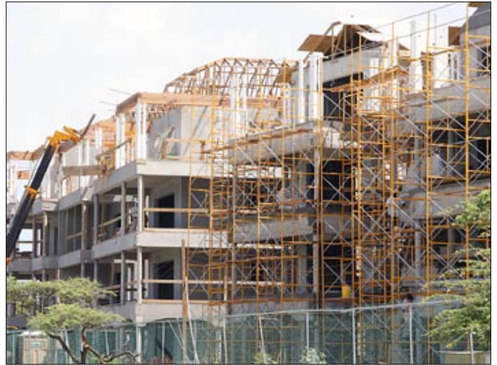
Construction of a new hotel at Pigeon Point
