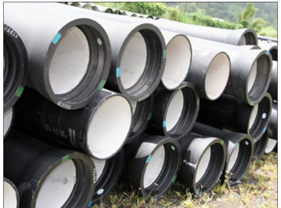
New 20" pipes for water distribution
