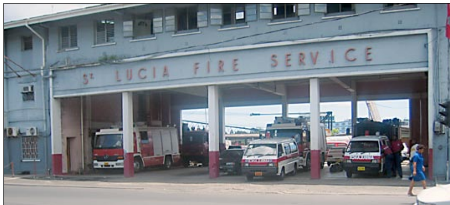
Castries Central Fire Station
