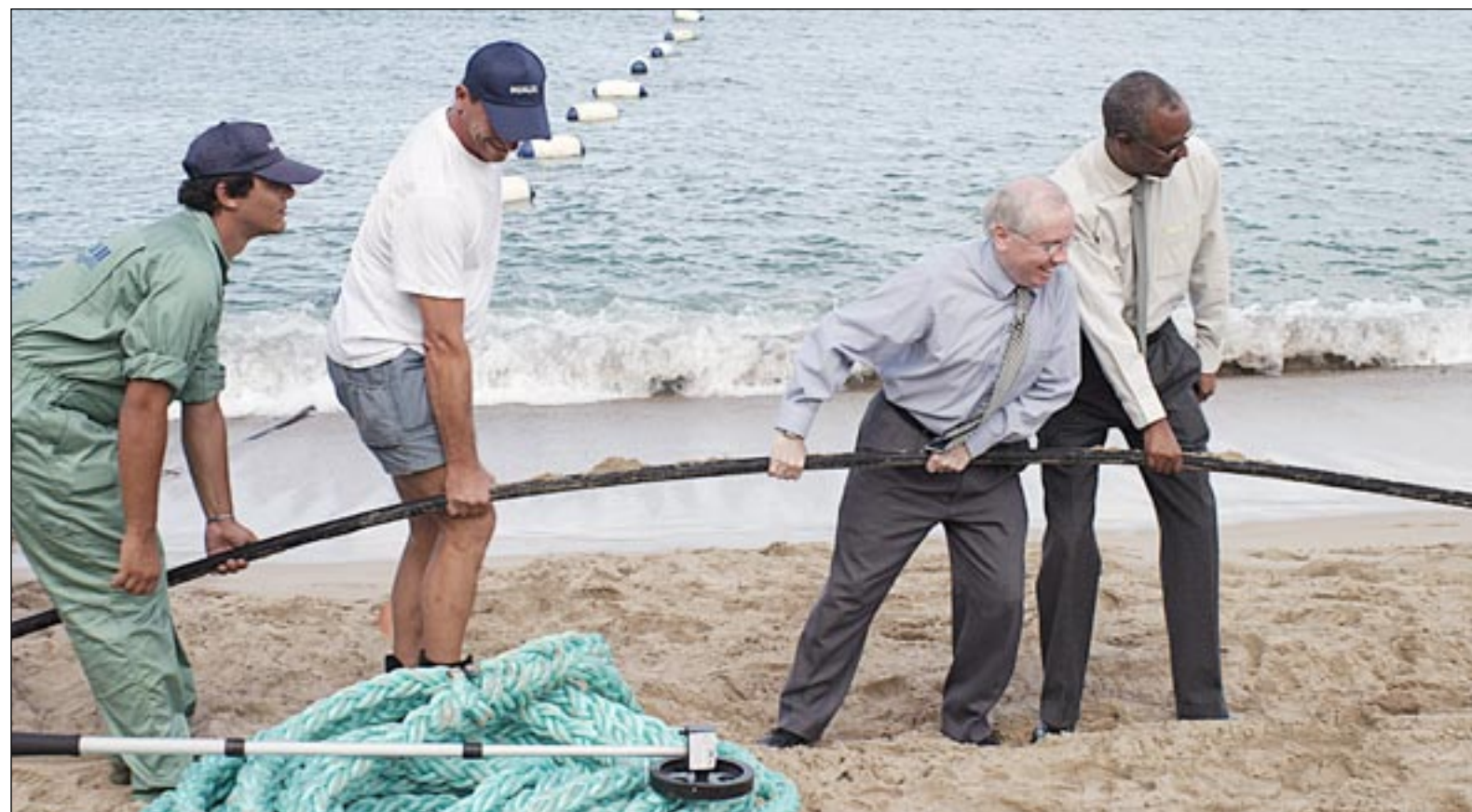
Broadband Cables being landed in Saint Lucia by Antilles Crossing
