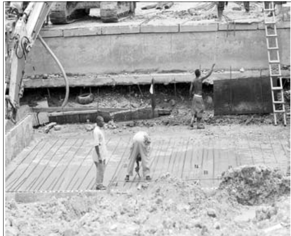
Flood mitigation works continue in Anse La Raye.
