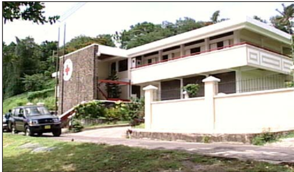
NEMO's Office in the Red Cross Building at Vigie, Castries
