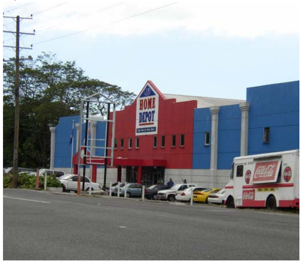
A facelift for commercial buildings, part of the new Government incentives.
