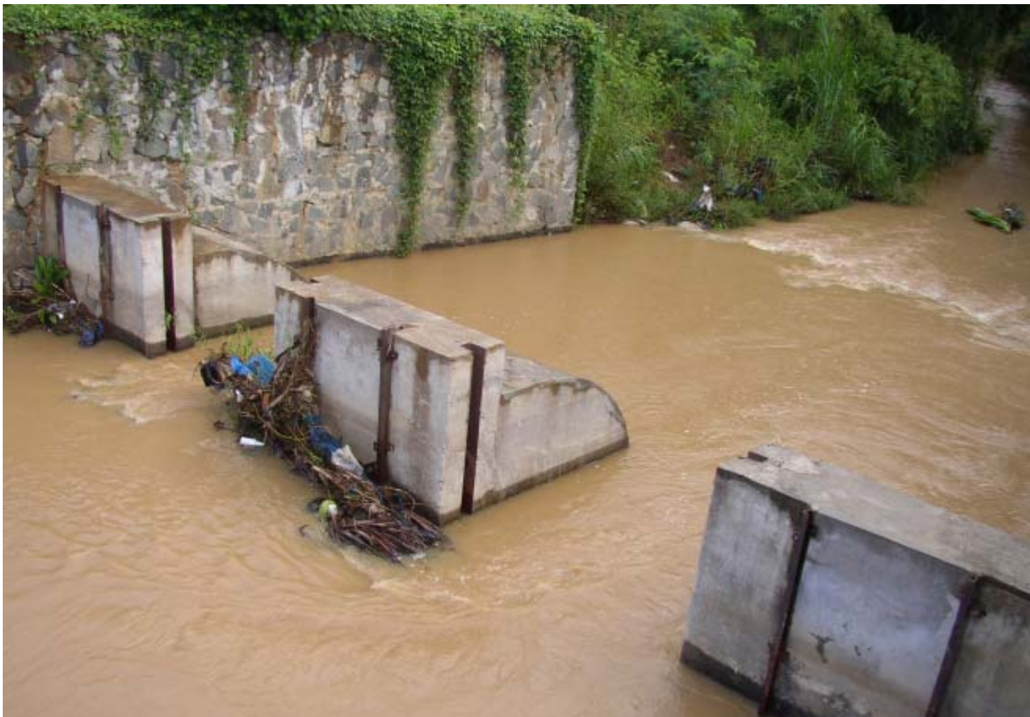
In-take Dam: part of the irrigation infrastructure in Cul-de-Sac
