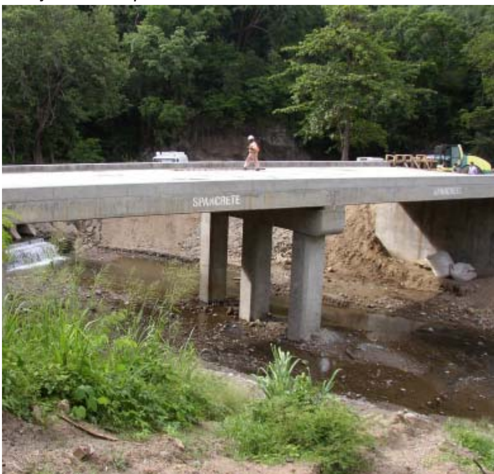
The new River Doree bridge under construction.
