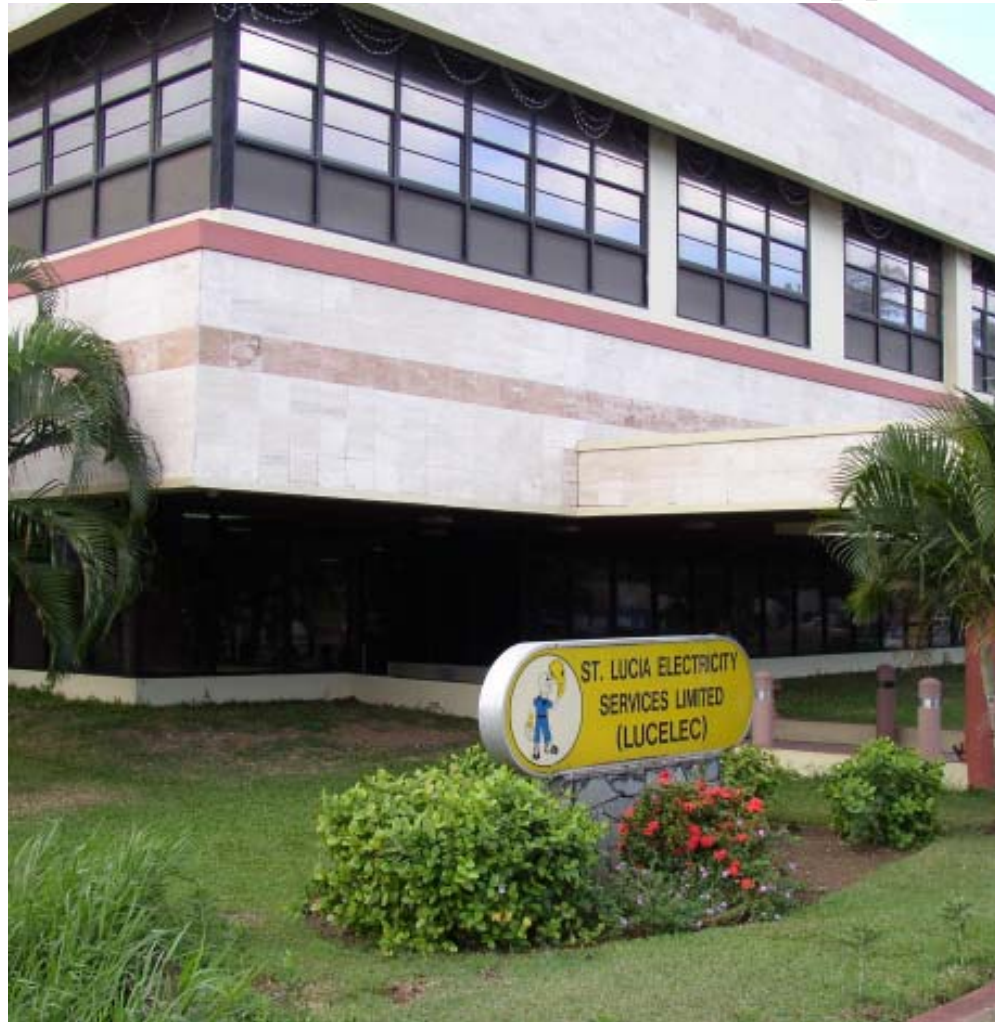
The head office of the St. Lucia Electricity Services Ltd. located at Sans Souci in the capital city, Castries
