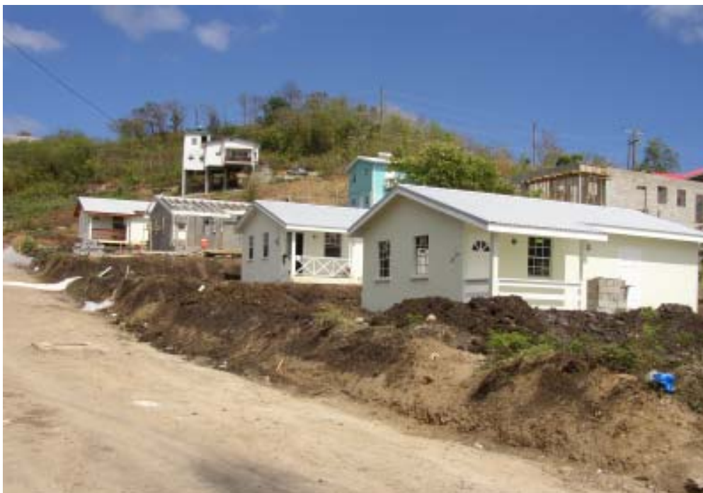
HOUSING THE NATION: homes under construction at Beausejour.
