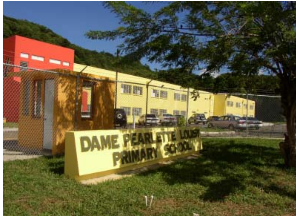
EDUCATION: Construction of new schools – an integral part of Government's modernization strategy.
