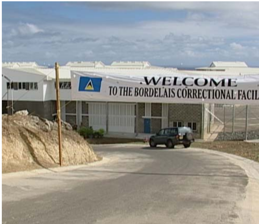
The infrastructure at Bordelais is built according to international standards.
