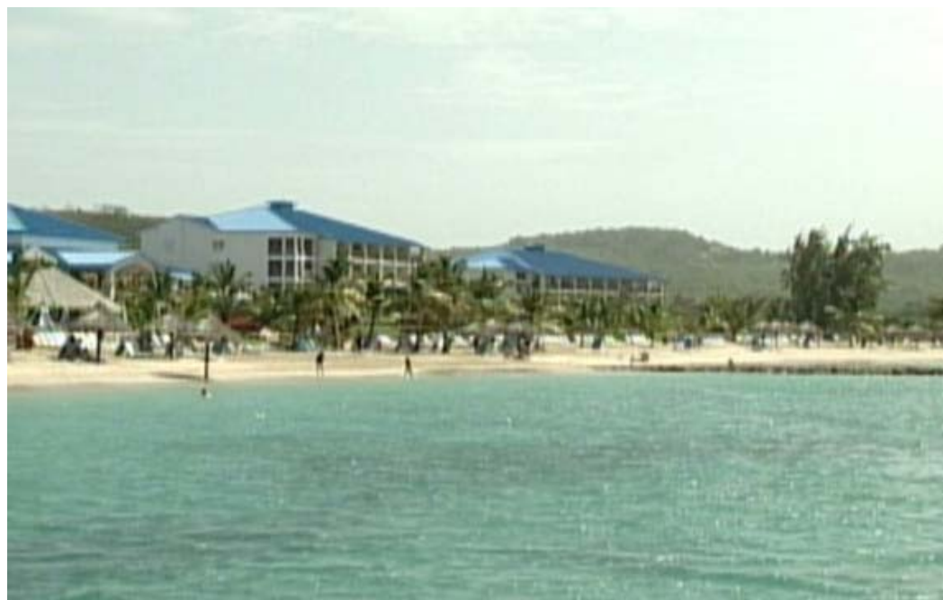
Hotels and resorts built near the shore can be easily affected by rising sea levels.
