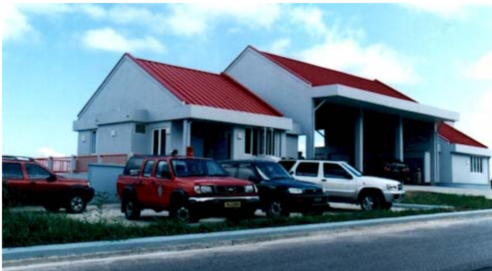
The newly constructed Dennery Fire Station with improved working conditions for fire officers and modern fire-fighting equipment.
