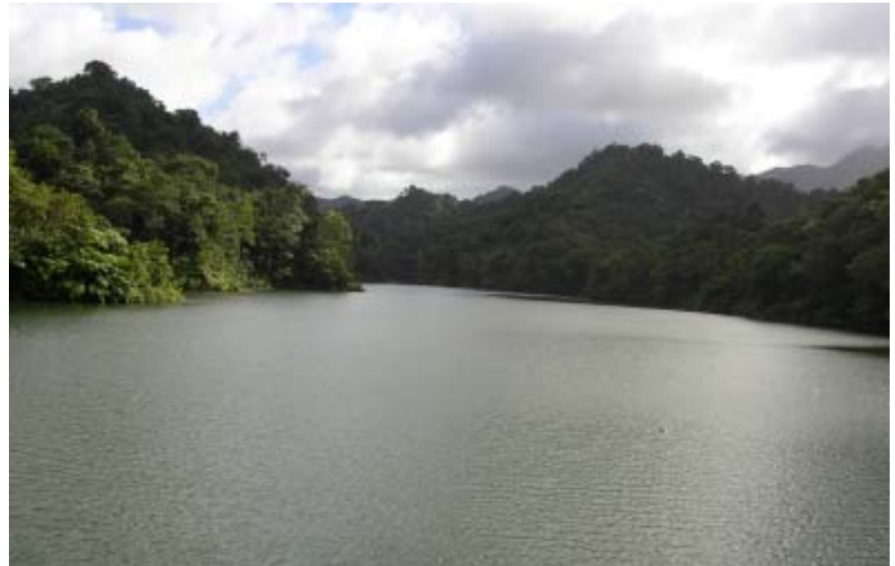
The John Compton Dam, located in the heart of the Roseau Valley: A storage capacity of 800 million gallons
