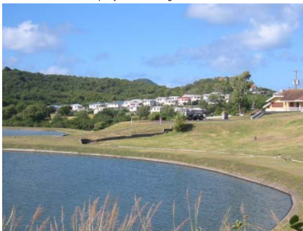
The sewerage treatment plant - a critical component of WASCO's operations
