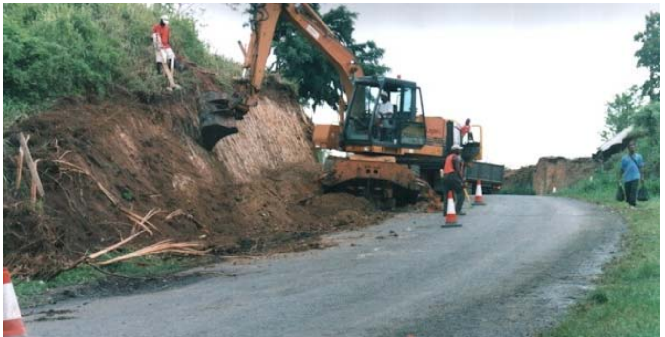
Excavation work along a Choiseul section of Soufriere-Vieux Fort highway.
