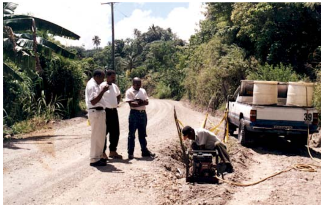
Officials on site at the Tet Chimen Water Development Project
