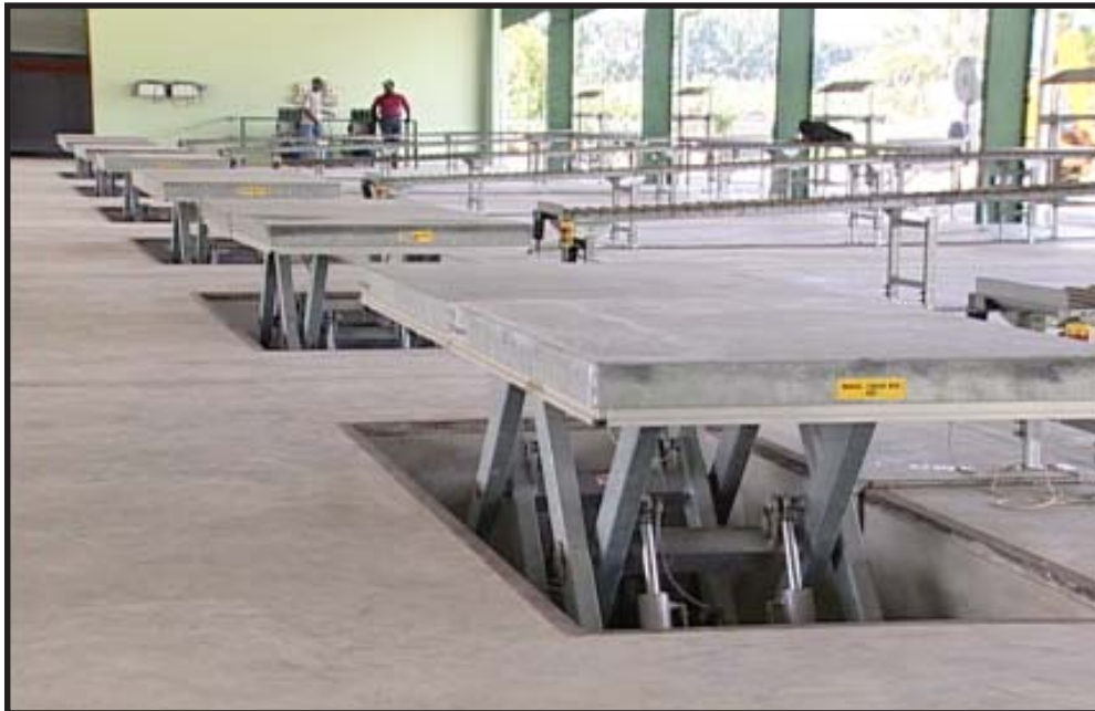
Hydraulic Lifts at the Odsan Inland Reception Distribution Centre
